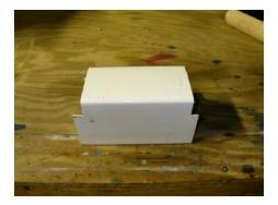
4. Make a template for your side pieces by using a small piece of gutter material and carefully tracing along the **inside** wall of the gutter onto your template material. I use a piece of the same vinyl siding that will be used to make the actual side pieces. Try to make the template fit as closely as possible inside the gutter as this will make gluing the side pieces much easier. Carefully draw and cut out the side pieces for the filter.
